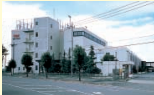
CMK PACKAGE TECH headquarters in Technical Center Plant
