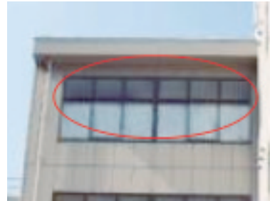
Heat-shielding, light-blocking netting mounted on the windows
