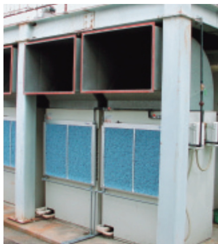
water sprinkler system for outdoor units
